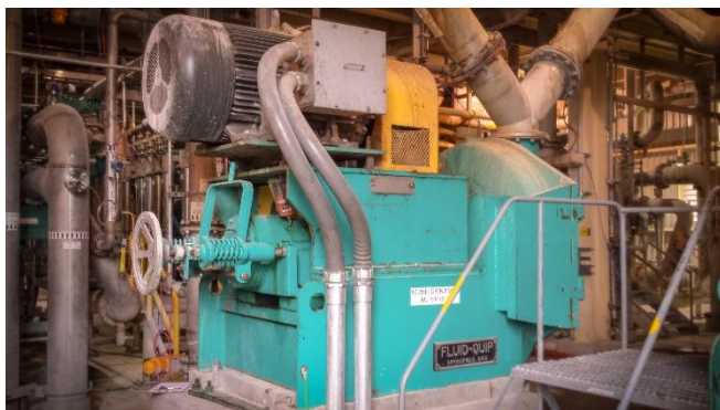
Fig.1 Large Direct Driven Wet Corn Mill
